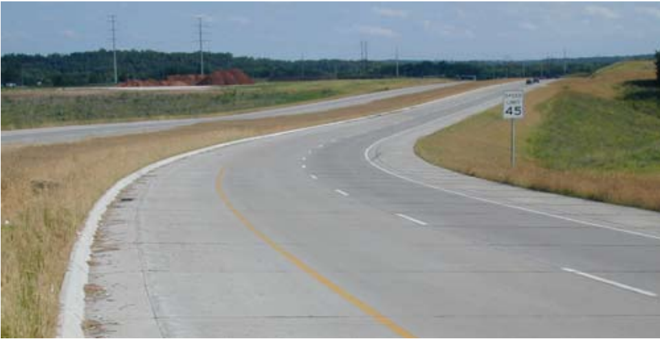
The new Highway 150
